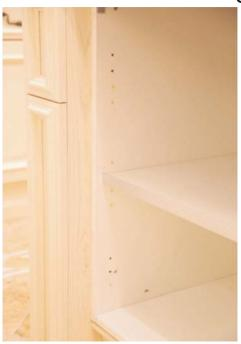
10.2.2 Make sure the door is in line with the bottom part of the cabinet, then fix it to the carcase
