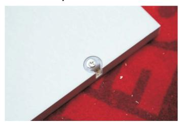
Fix the shelves and the shelves support with the screw on the plastic insert.
