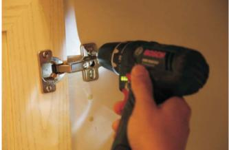
10.2.3 If the doors are not in the same line after fixing, then we need to adjust the doors
